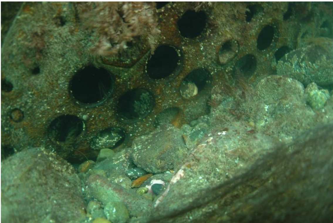
Figure 6.8 Boiler tubes (Source: C. Holden)
