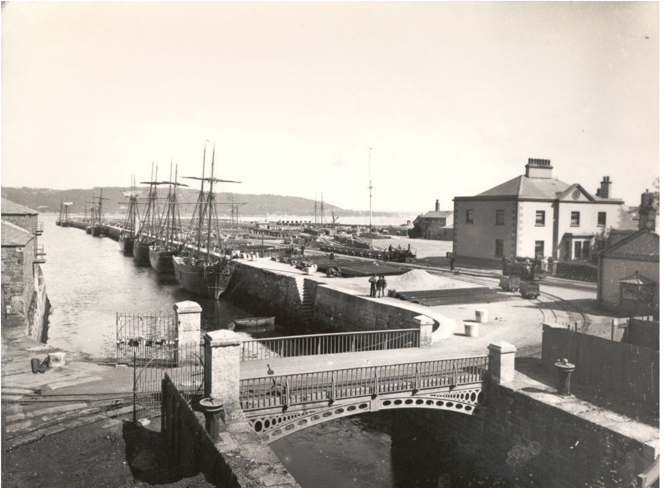
Fig. 4 Penrhyn Port, Bangor ©Gwynedd Archive Service
