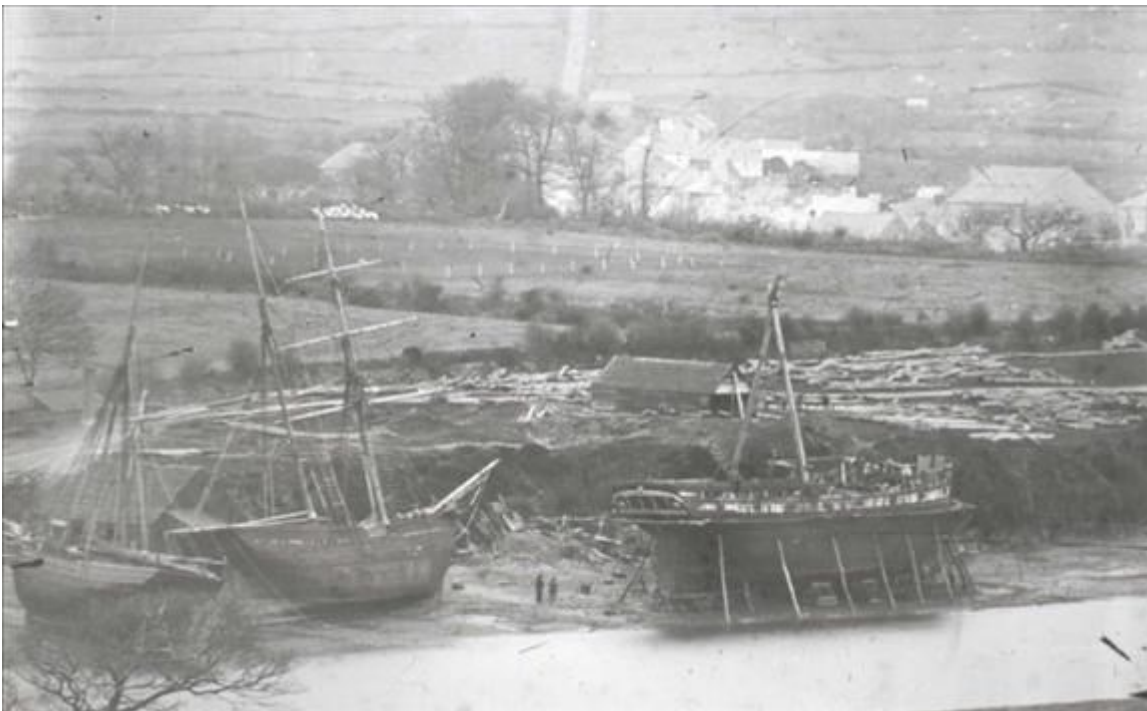
Fig. 1 Cardigan Ship Building 19 th century
