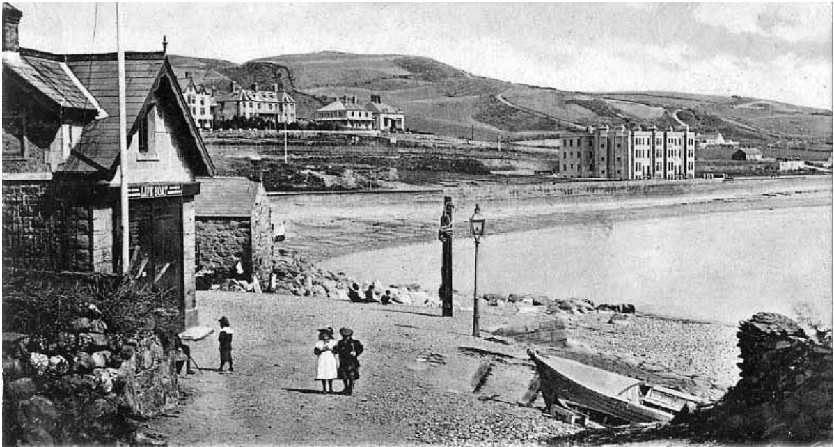
Criccieth Lifeboat Station The post for securing the shoreside end of the towing out warp with the "lizards" attached can be seen.
